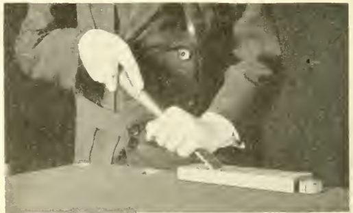
Fig. 22. Whetting the Beveled Side of a Chisel.
